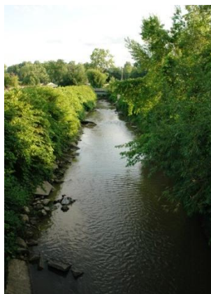
West Creek, Channelized
