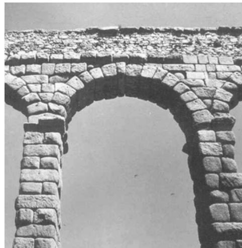
H. Arcuated Construction (Roman Arch above)
