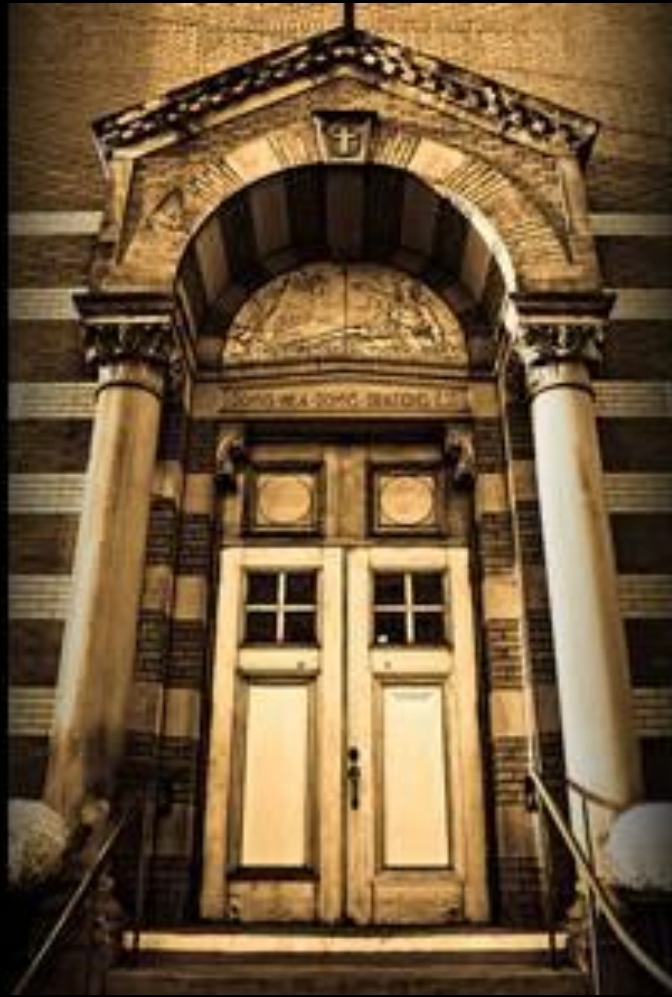
Entry, Catholic Church in Pittsburgh, Pennsylvania
