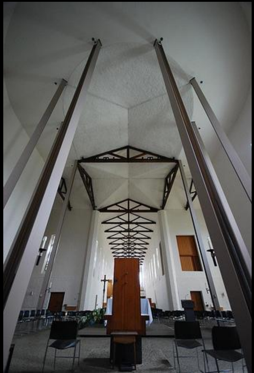
Looking towards Sanctuary
